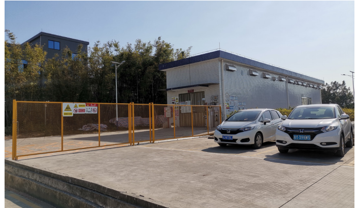
In our China tannery, we installed a fence to prevent unauthorized outsiders from entering the Hazardous Chemical Warehouse
