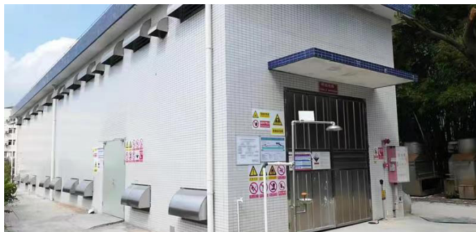
In our China tannery, we store hazardous chemicals separately at the Class A warehouse, which was built in line with the Code for Fire Protection Design of Building, aiming to guarantee the safety of the chemicals
